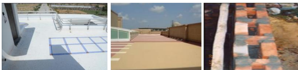
Figure 5: Use of High HRI coat on roof top and Use of Cavity wall on the western side of the buildings
